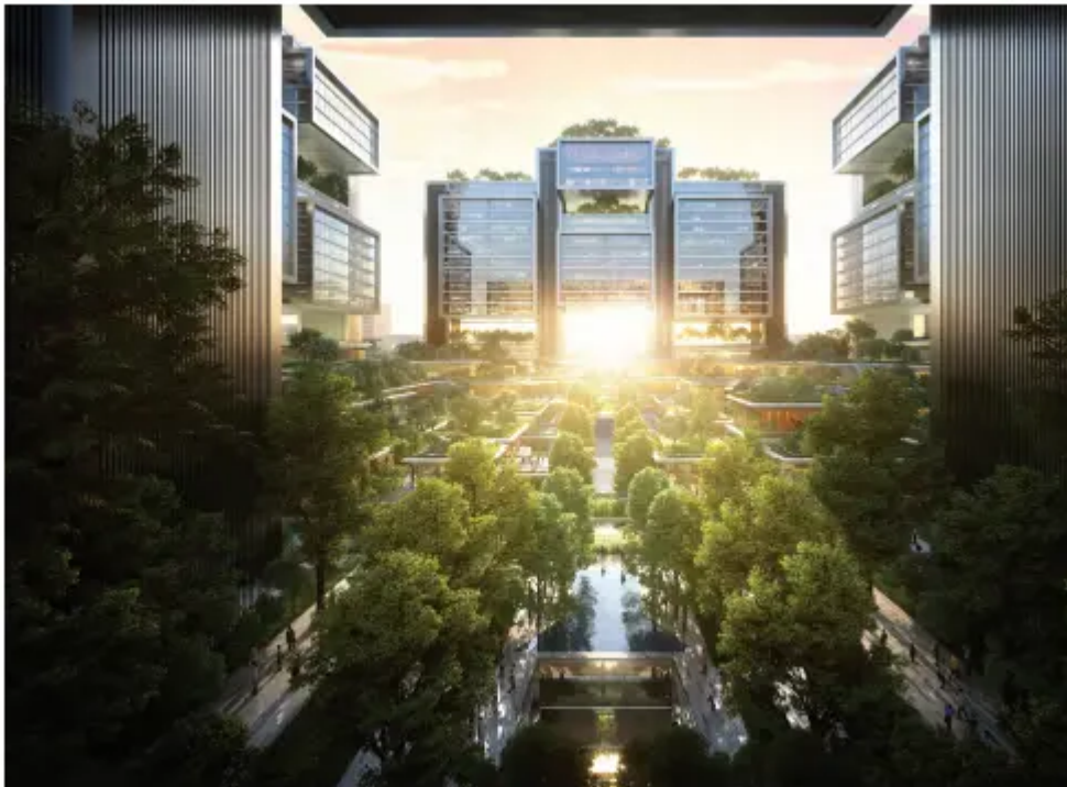
A series of office towers acting as 'gateways' to the urban center.
