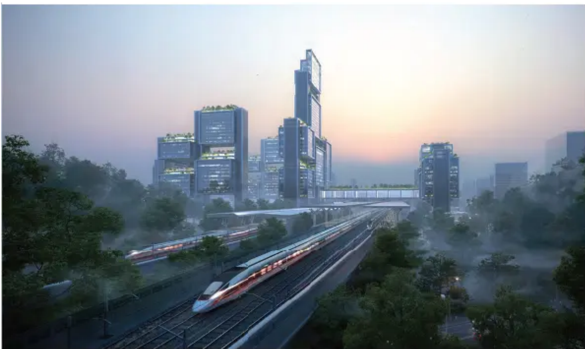
A contemporary urban center with an integrated and sustainable transport hub at its heart.
