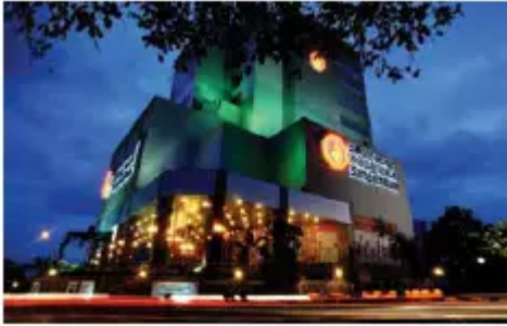
Sampath Bank Head Office.
