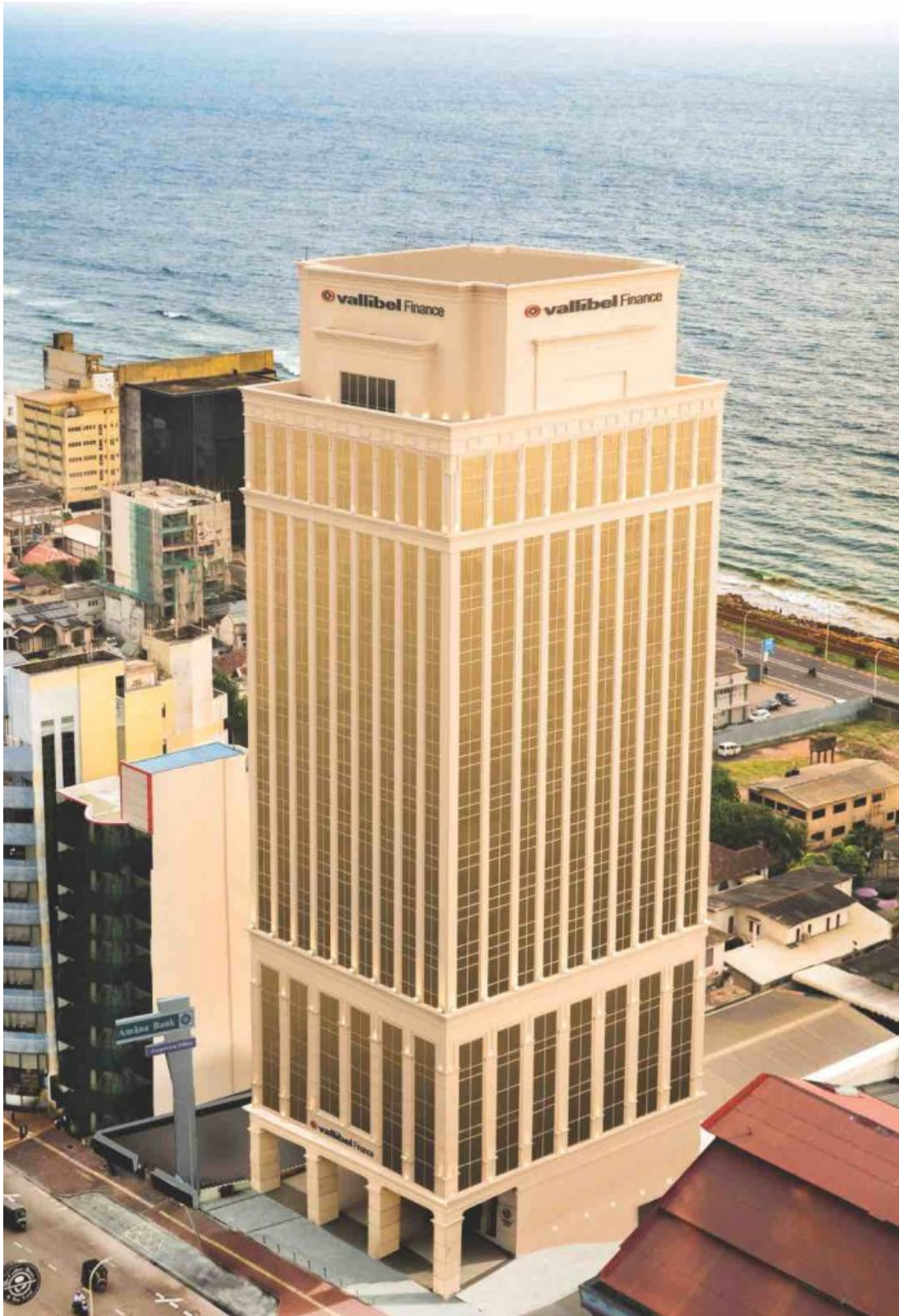
The impressive Vallibel Finance corporate office building is located in Colombo 3.
