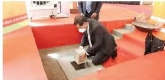
Ranjith Kodithuwakku, Chief Executive Officer/General Manager laying the foundation stone at the building site.
