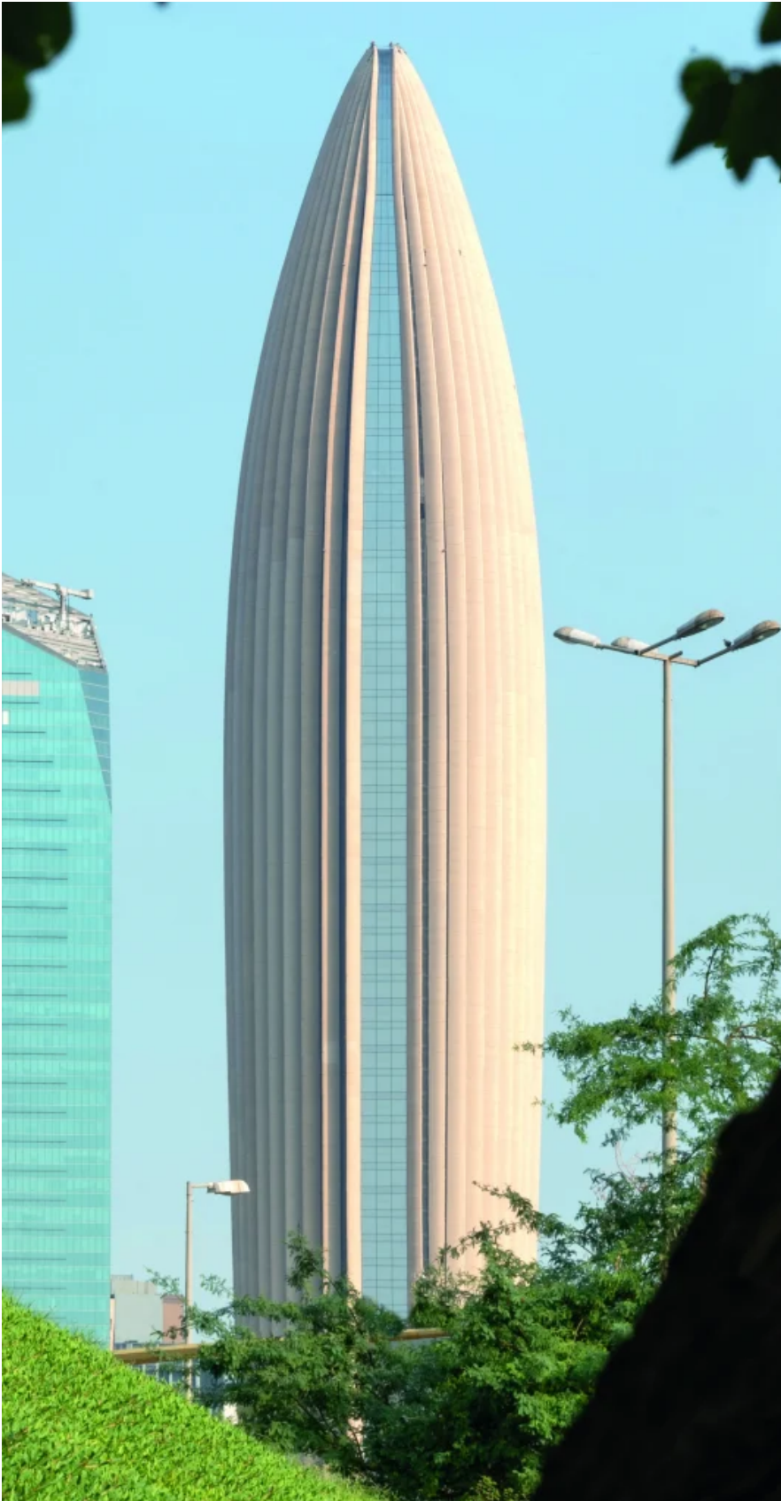
Exterior view of the National Bank of Kuwait. The design combines sustainable features and structural innovation, providing an energy efficient passive form, shielding the offices from the extremes of Kuwait's climate.
