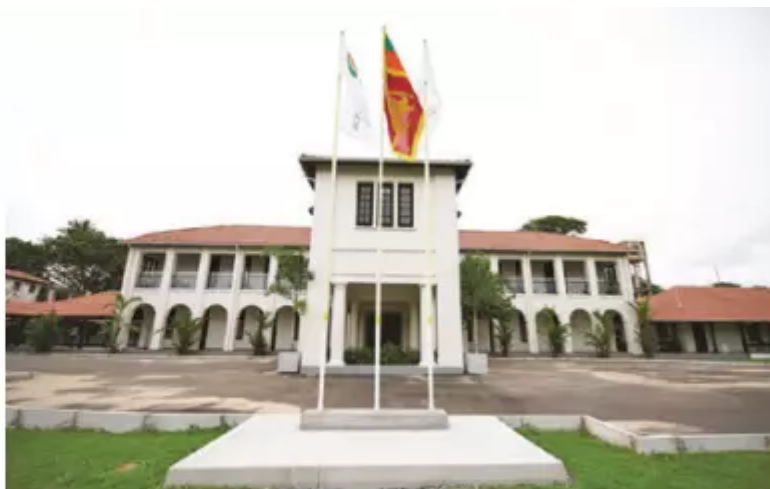
The renovated Joseph Fraser Memorial Hospital.
