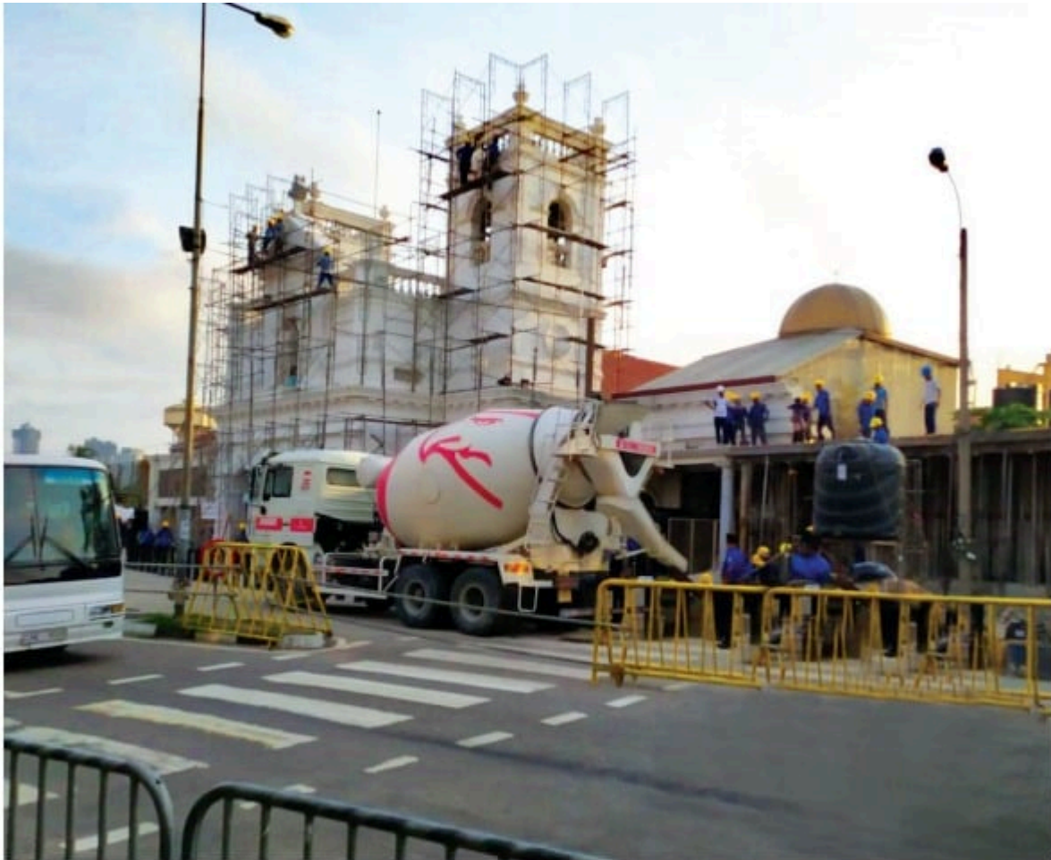
St. Anthony's Church, Colombo 13 under restoration.
