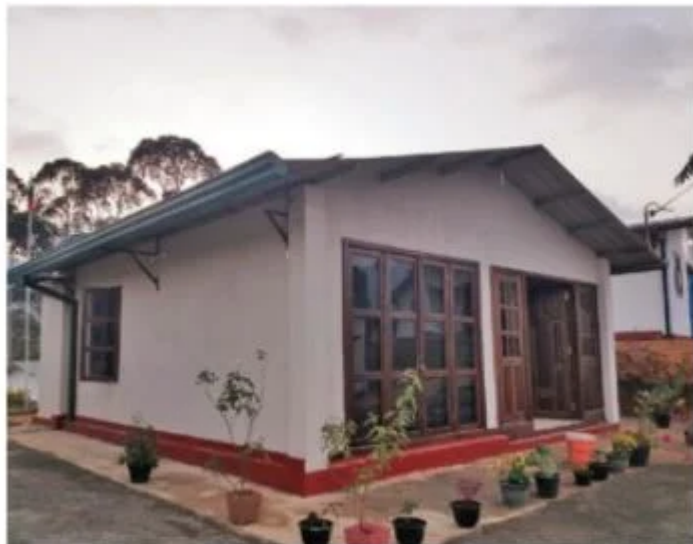
One of the houses built under the Indian Housing Project.
