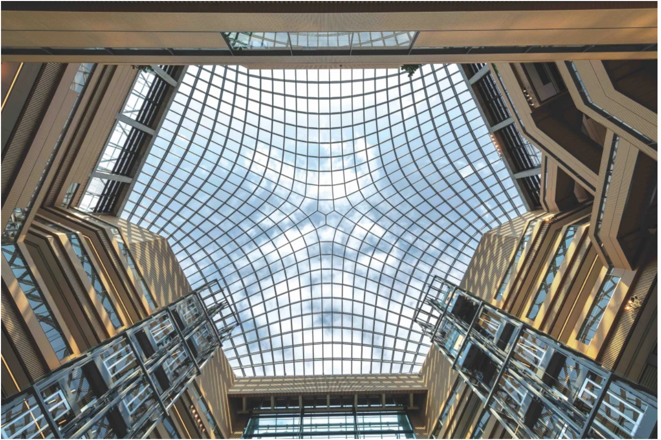
View of the glazed roof geometry. Triple glazed panels are cold bent into place onto an optimised lightweight steel grid shell structure.
