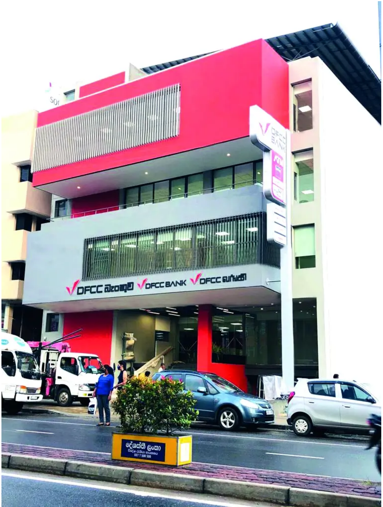
Rooftop Solar Power System installed at DFCC Bank Kurunegala Branch.
