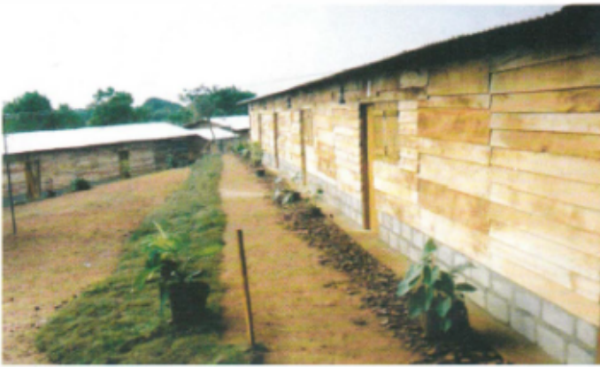
A temporary housing project where 150 homes were constructed in Tissa.
