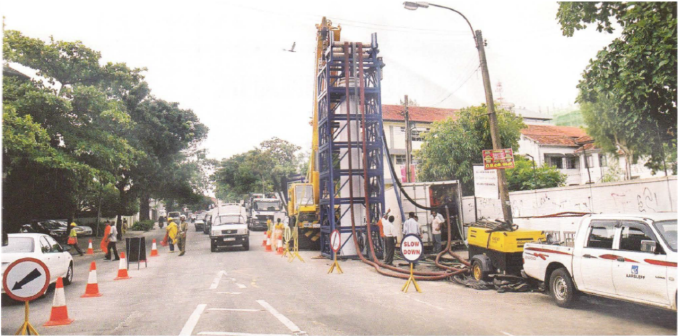
Site of works at Sir James Peiris Mawatha, Colombo
