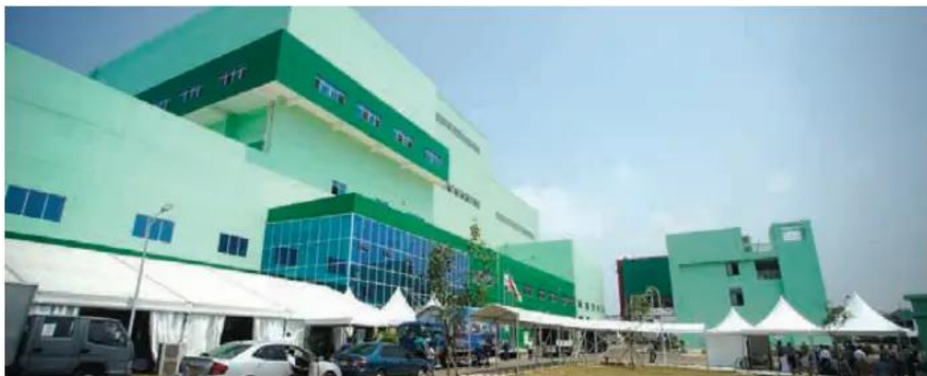
Sri Lanka's first Waste-to-Energy Power Plant by Aitken Spence's Western Power Company.
