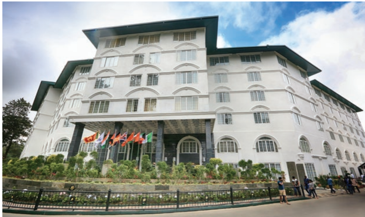
The elegant façade of Araliya Green City
